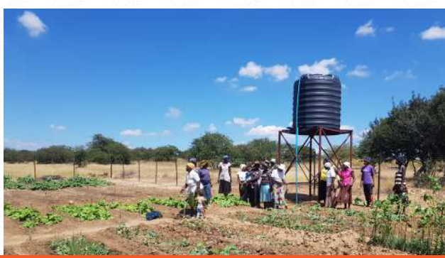
Water storage facilities and water reticulation system through installation of water taps in the nutrition garden has lessened the burden of work for women to water plants in the nutritional garden, women can now save time to engage in other productive economic activities outside of the garden
