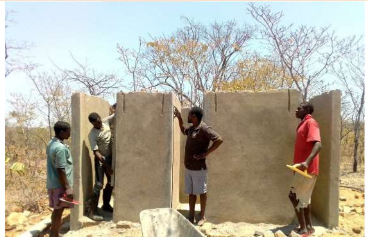
Toilet constructed by building vocational skills at Mutiwegora
