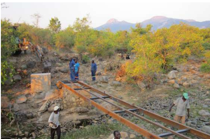
The process of community footbridge construction
